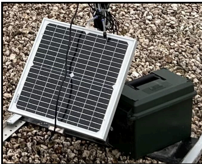
Figure 12: BluBird power supply system: solar panel and backup battery.
